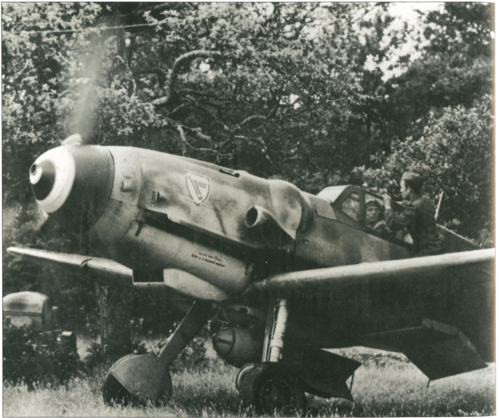
Messerschmitt Bf 109 G-5/R1 possibly with Major Heinz Bär in cockpit while attached to Stab JG 3 "Udet" in June 1944. This aircraft is fitted with R1 kit (ETC 500 IXb bomb container) carrier SD 500 fragmentation bomb. [Deutsche Museum]
